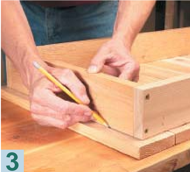
3 LAY THE FRAME on the top boards and lightly trace the frame shape so it's easy to see where to drill holes. Space the top boards with about 1/16-inch gaps between them.
